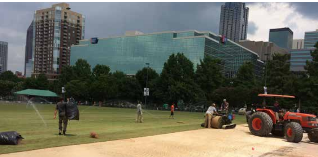
Crews install new sod on the surface of Centennial Park after completing work on an innovative sand-capped root zone to promote better drainage and minimize grass damage during rain events.
