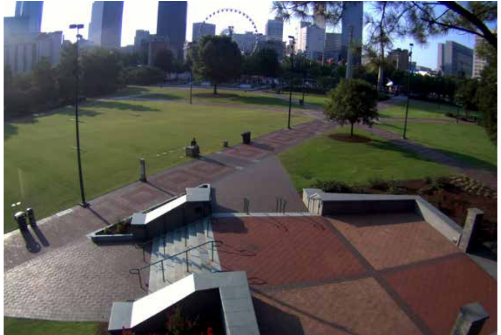
Once installed, the sand-capped section of the lawn looks identical to the rest of the park's grass-covered areas. The system of drainage tiles, gravel and sand mixed with an inorganic soil amendment is hidden beneath the sod.
