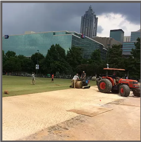
Park reconstruction underway
