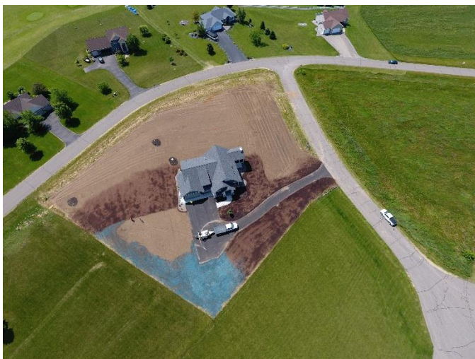
Installation June 26 th
