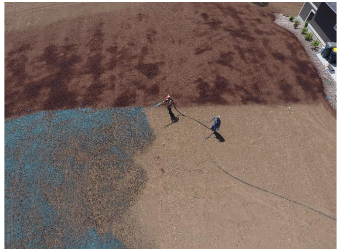
Installation June 26 th
