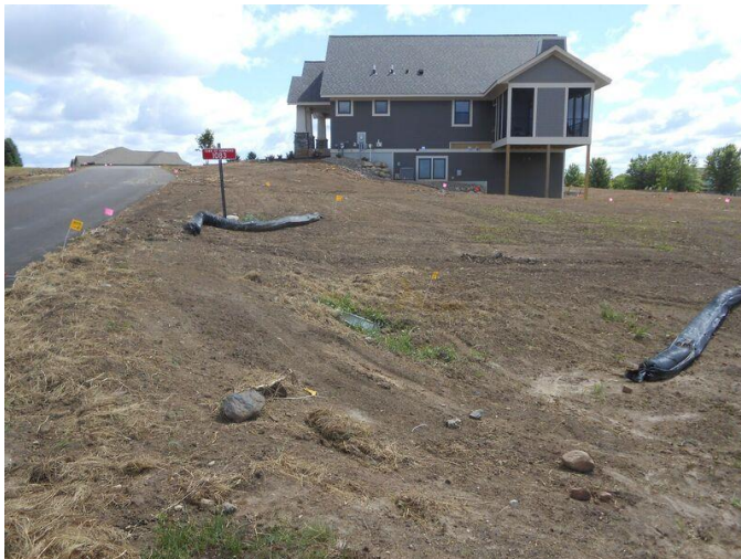
Installation June 26 th
